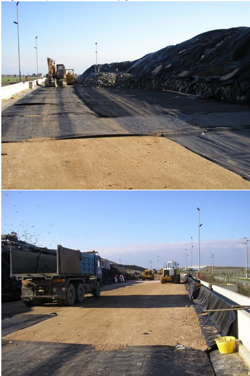
Image3 3 & 4: Preparation of foundations and laying of basal liner
