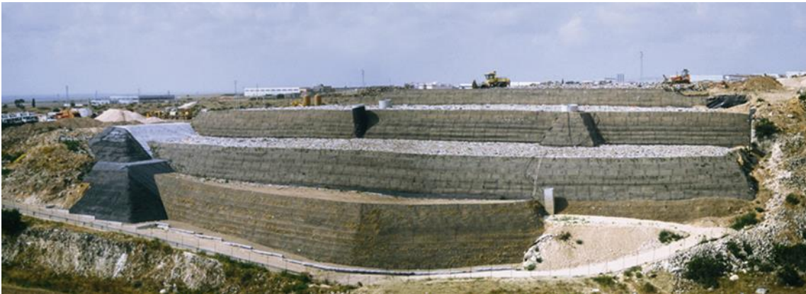
Image 2: Pariti 2 landfill, Foggia after consolidation using Frisoli technology
